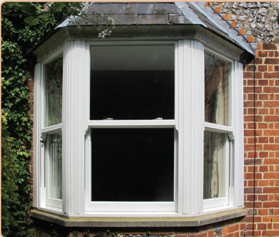
Mechanically Jointed Sashes
